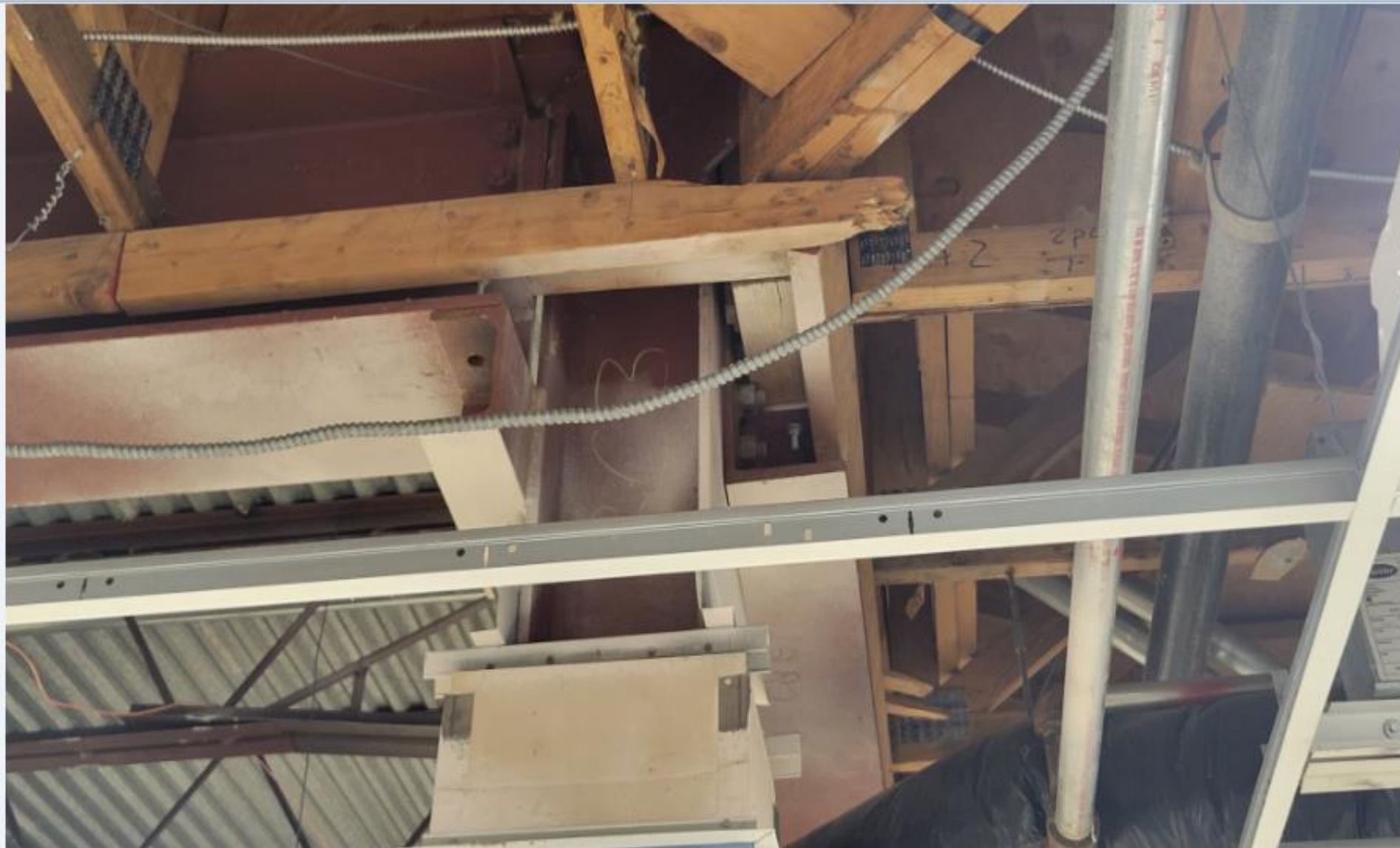
Structural Repair and Wood Blocking
