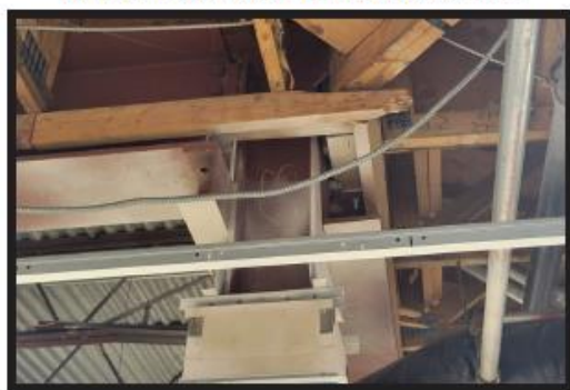
Structural Repair and Wood Blocking.
