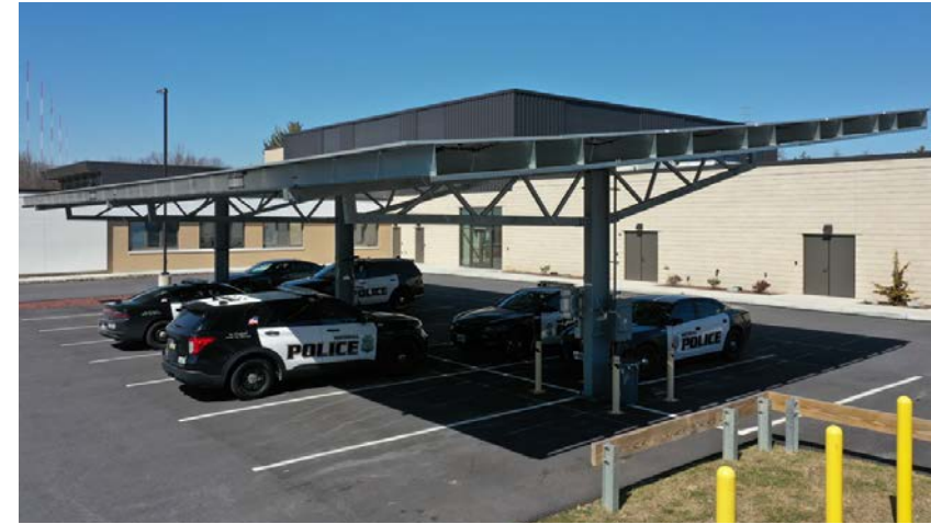
Whitehall Township Police Station
