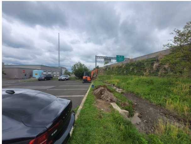
Photograph 3 – Looking South towards Test Pit Locations TP-104 & TP-105
