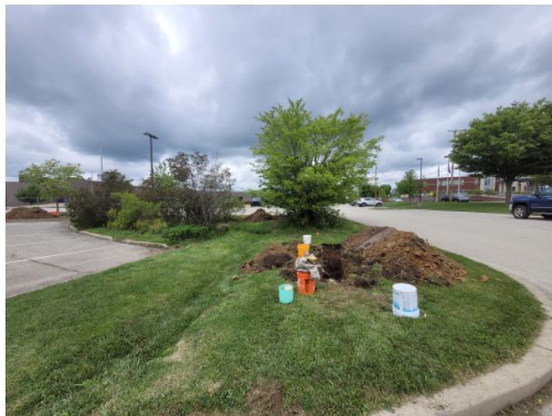
Photograph 1 – Looking West towards Test Pit Locations TP-101 & TP-102
