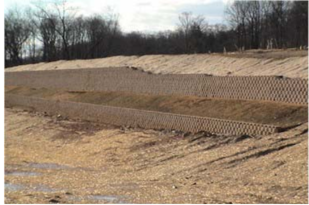
Figure 5.1-6. Woodland removal for steep slope development with retaining walls
