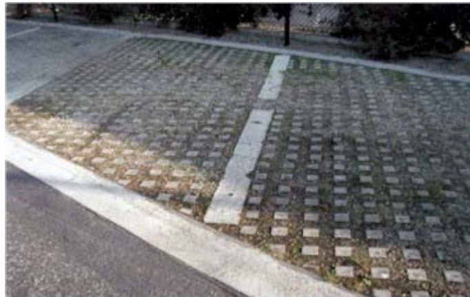
Figure 5.10-2 Overflow parking using permeable pavers
