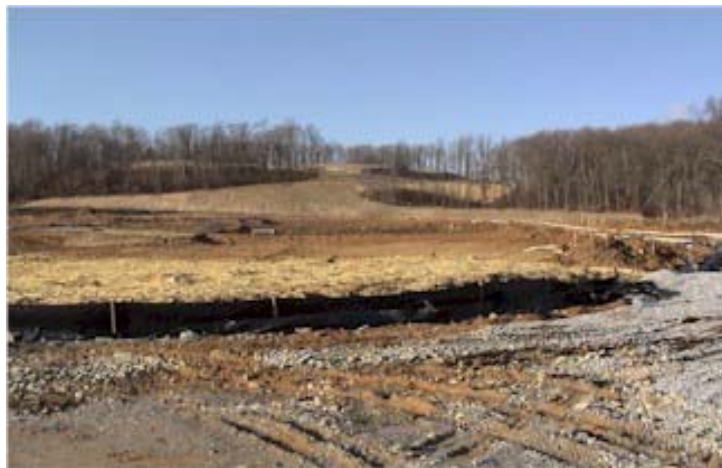
Figure 5.7-1 Example of development with site compaction of soils
